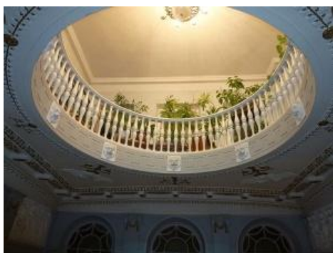
Fig. 8. Interior view of the house the merchant of the First Guild I.I. Smirnov
