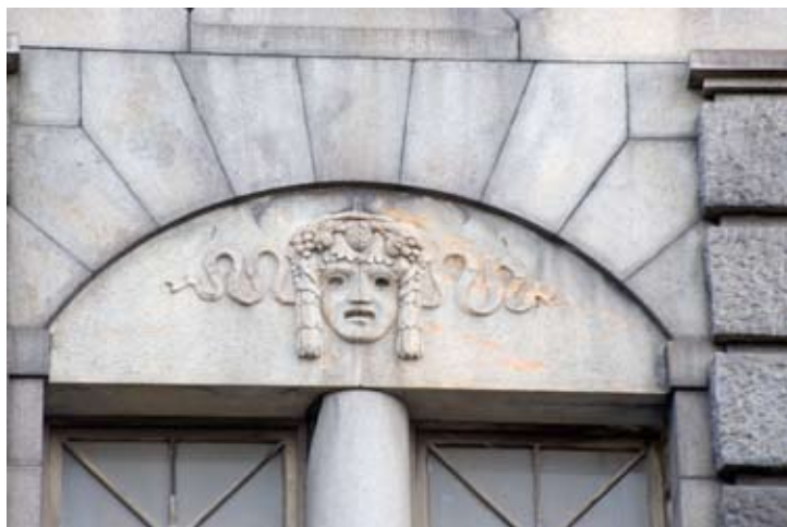
Fig. 6. Second Mutual Credit Society Building. Window pediment, decorative detail. Photograph: William Brumfield (2/1/2017)
