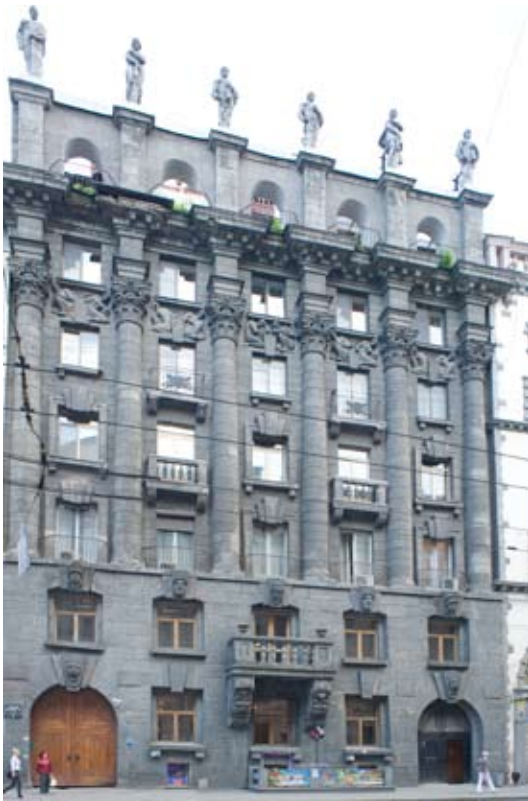
Fig. 14. St. Petersburg. K. I. Rozenshtein apartment building, Kamennooostrovskii Prospekt, No. 35 & Bol'shoi Prospekt, No. 77. Photograph: William Brumfield (30/5/2013)
