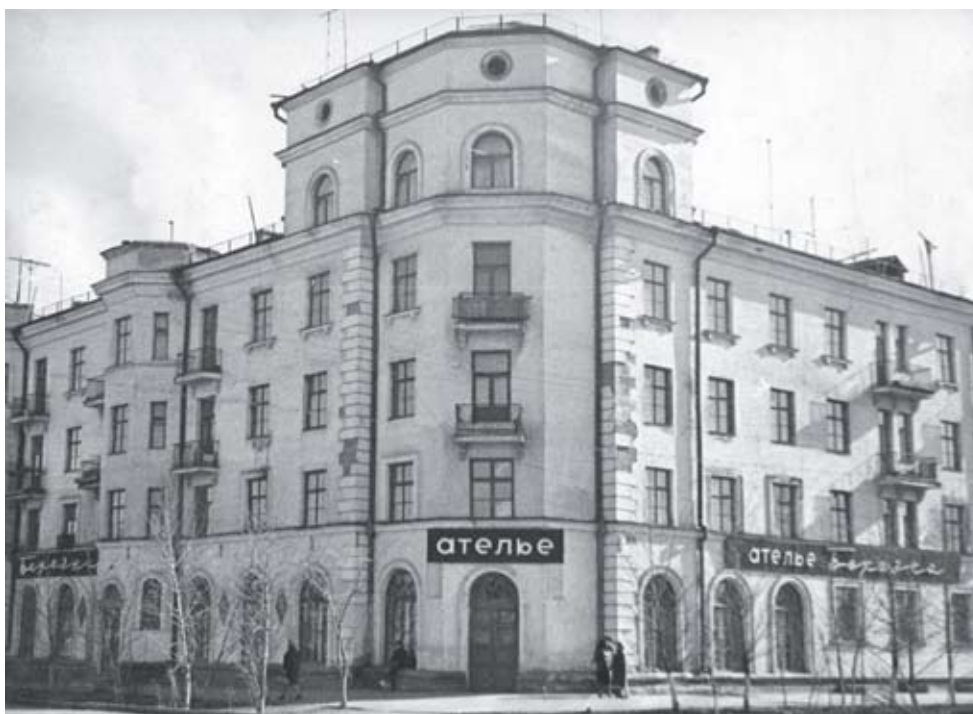
Fig 1. Chernogorsk town, Sovetskaya / Dzerzhinskogo Streets, residential house “the Sputnik”. Photo of 1960s. 2
