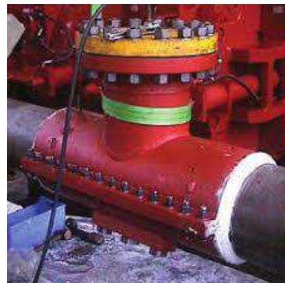
Рисунок 8 – Grouted tee one branch connection
