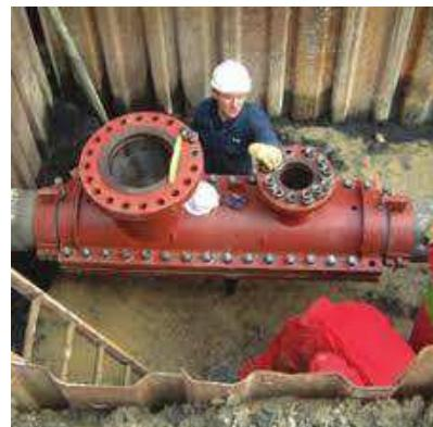
Рисунок 9 – Grouted tee double branch connection
