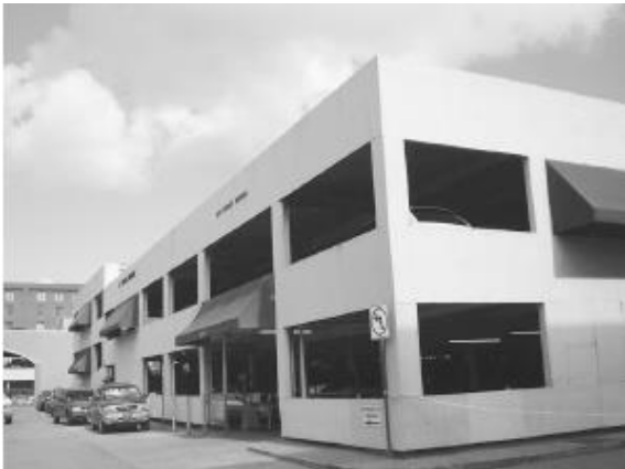
Figure 6. Parking garage in the Ellis square
