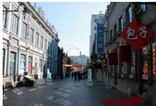
Figure 19. The restored street
