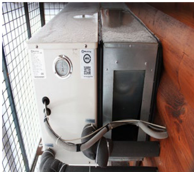
Fig. 2. Photo of the mixing chamber (patent No. 185689) and VTH installed in a low-rise residential building
