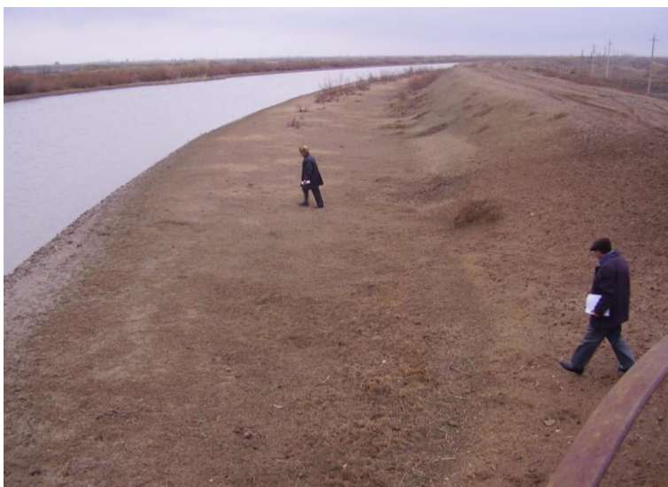
Fig. 4. General view of the Mirishkor canal in PK150 station
