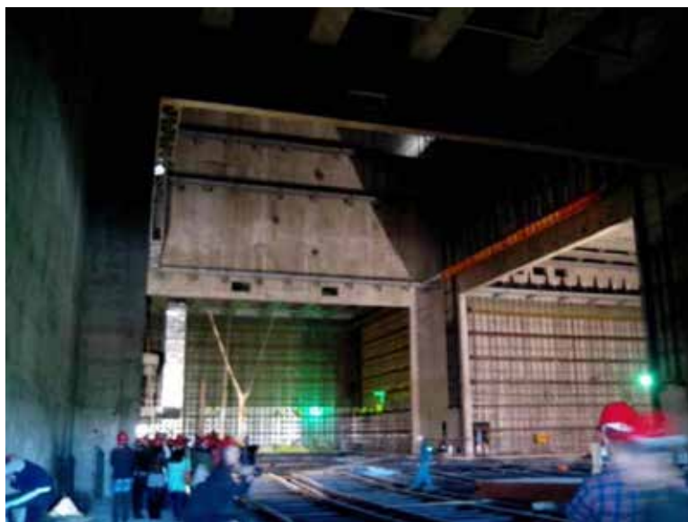
Fig. 5. Construction works inside the stage space. Author's photo, October 2014
