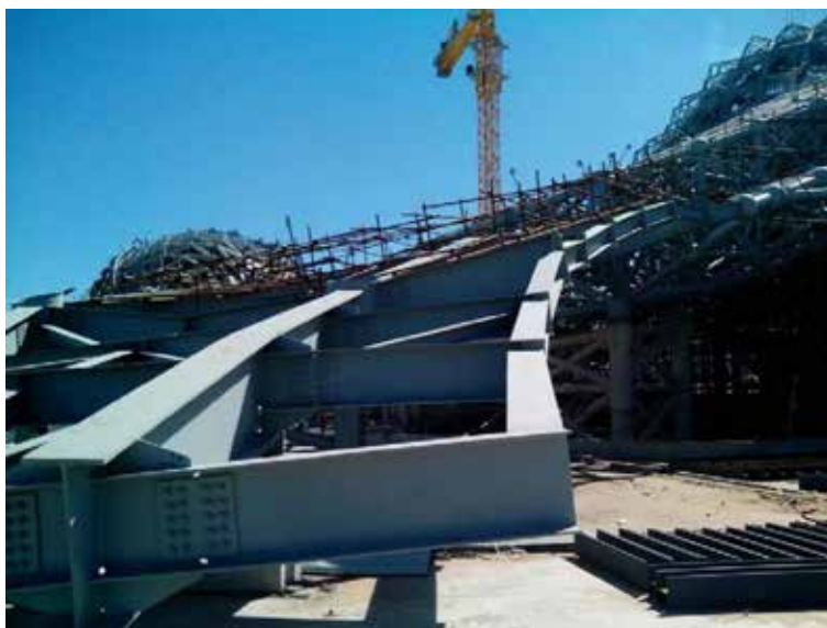
Fig. 13. Curvilinear form structure of I-section elements. Author's photo, October 2014
