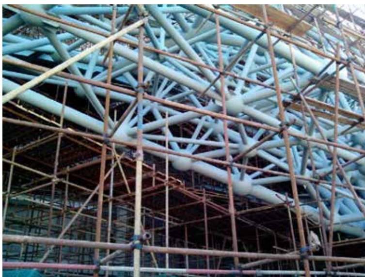
Fig. 12. Ball joint connections. Author's photo, October 2014
