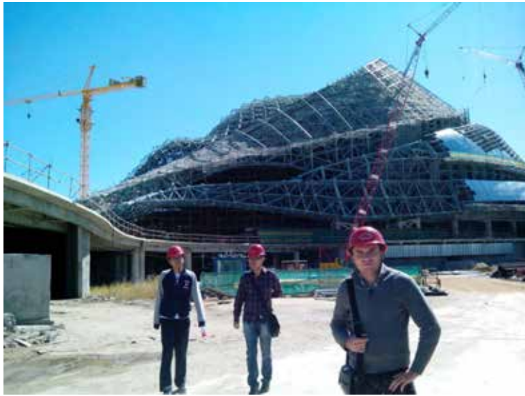
Fig. 10. Harbin Opera House construction process. Author's photo, October 2014
