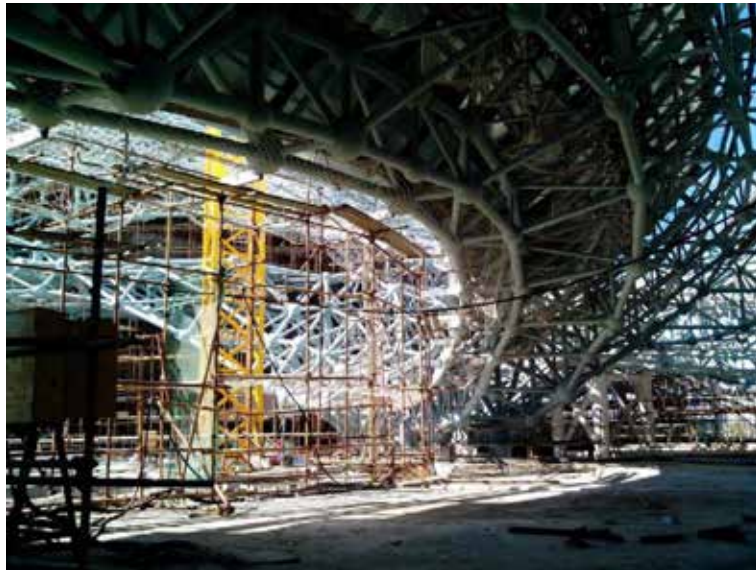
Fig. 11. Inclined arch structure using straight elements. Author's photo, October 2014
