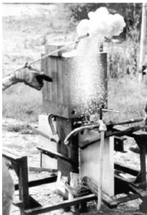
Fig. 3. Aluminum busbars welding with the method by ERICO
