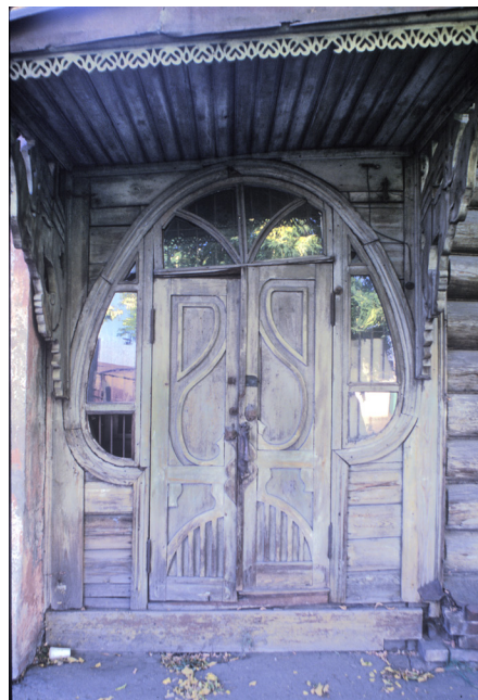
Fig. 15. Omsk. Log house, Michurin Street 48. Style moderne doorway. Photograph: William Brumfield (9/18/1999)
