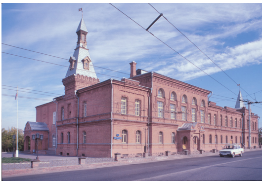
Fig. 19. Omsk. City Council (Duma) Building. Photograph: William Brumfield (9/18/1999)
