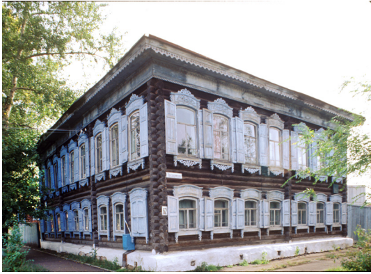
Fig. 4. Tara. Log house, Aleksandrovskaya Street 62. Photograph: William Brumfield (9/17/1999)
