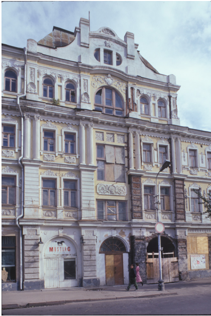
Fig. 25. Omsk. Kristall-Palas (Crystal Palace) Cinema Building. Photograph: William Brumfield (9/15/1999)
