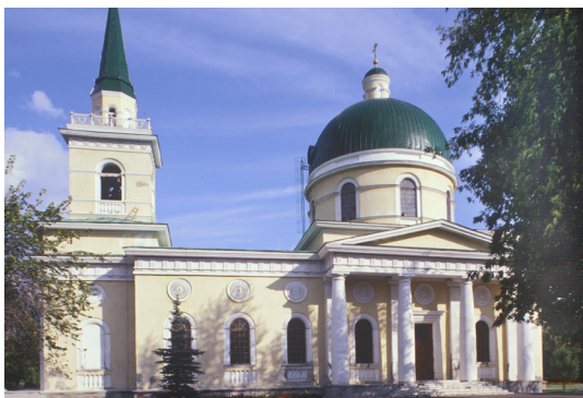
Fig. 11. Omsk. Cathedral of St. Nicholas. South view. Photograph: William Brumfield (9/15/1999)
