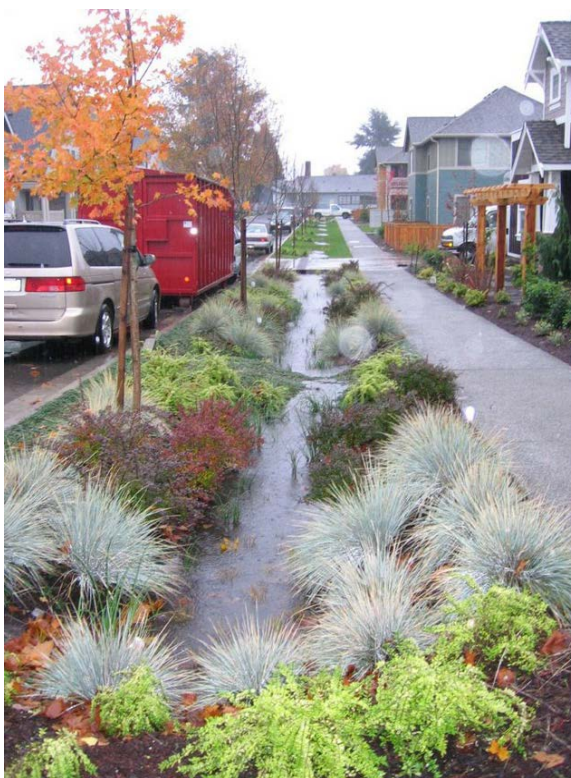
Fig.3 - Purification and reduction of storm water using plants and soil (Seattle, USA)
