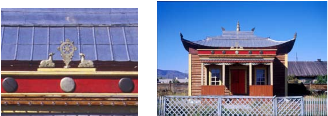
Fig. 37. Gusinoozersk. Tamchinskii datsan, wooden temple (Dugan Aiusha), pediment with figure of Dharma wheel (Eightfold Path) (a), Gusinoozersk. Tamchinskii datsan, wooden temple (Dugan Aiusha) (b)
