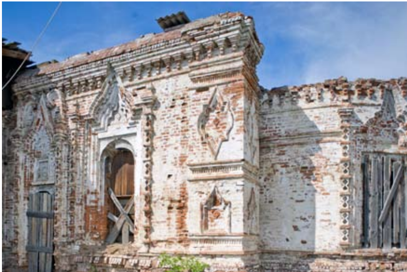
Fig. 31. Eniseisk. Church of the Trinity, south facade (under restoration), east corner, window surrounds and ornamental motifs
