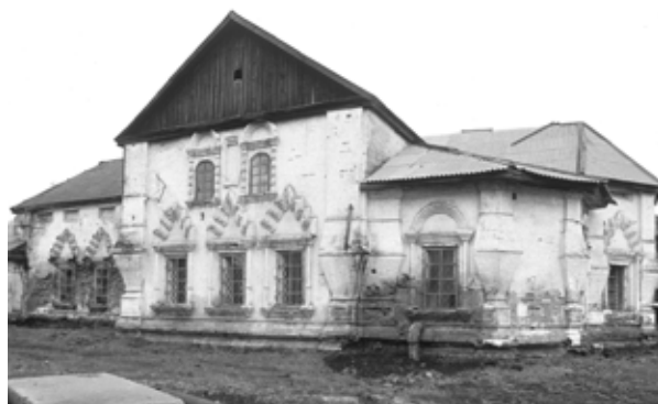
Fig. 1. Tobolsk. Church of the Miraculous Image of the Savior (Nerukotvornyi Spas), south facade. All photographs by the author
