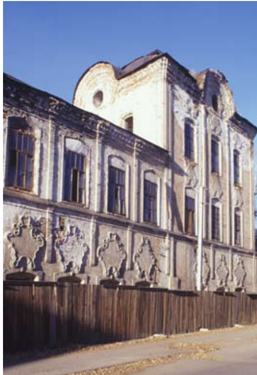
Fig. 18. Irkutsk. Church of St. Kharlampii (Archangel Michael), south facade
