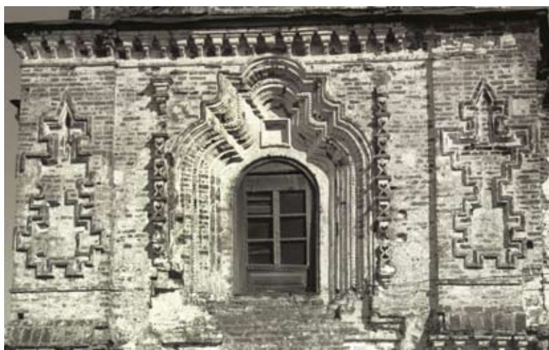
Fig. 28. Posolskoe. Transfiguration Monastery, Cathedral of the Transfiguration of the Savior, west facade, main portal with perspective arch
