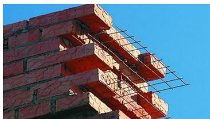
Fig. 12 Installation of stone and reinforced stone structures (developed b2b.by/montazh-kamennyx-i)
