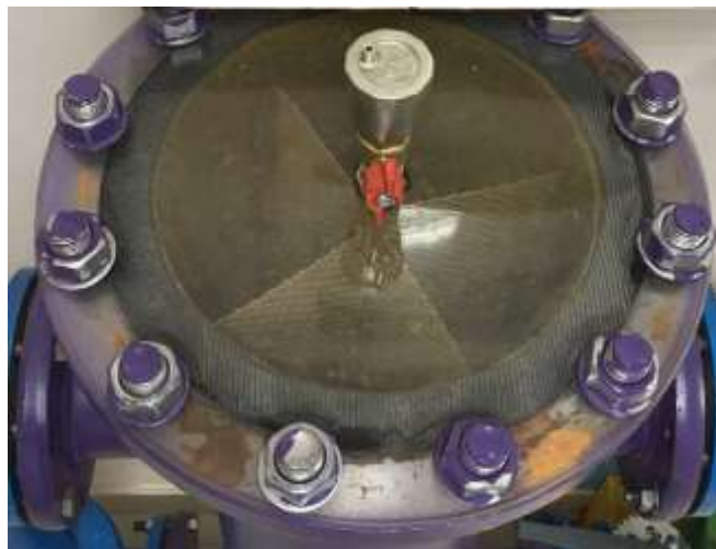
Figure 2. Separator of free air and gases.
