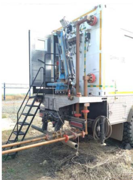
Figure 10—Mobile multiphase flow metering system
