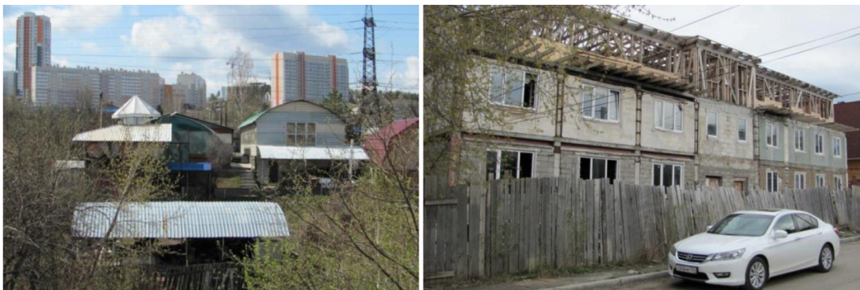
Figure 1. Buildings that do not meet regulatory requirements
