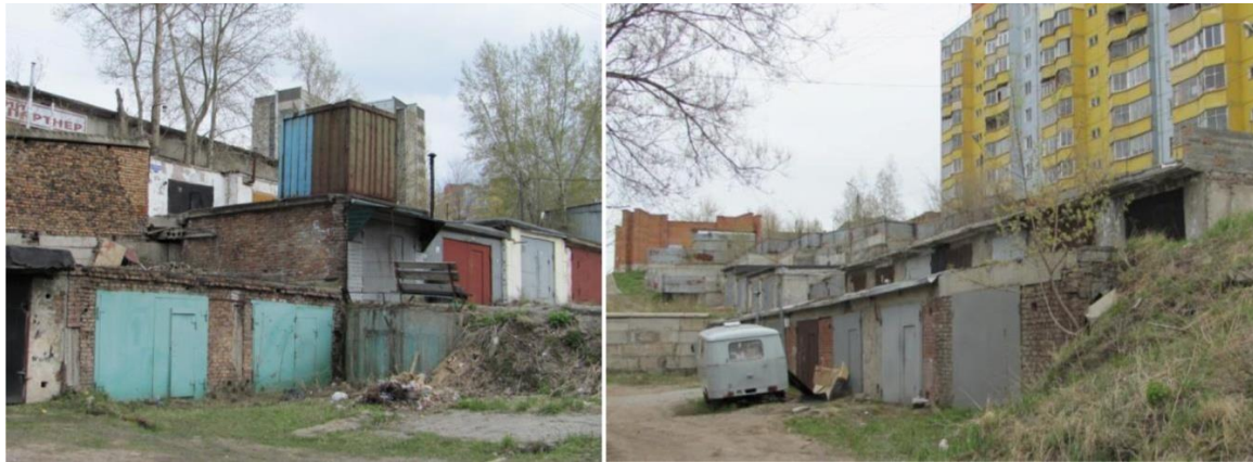
Figure 5. Garage arrays (Svobodny Prospekt)
