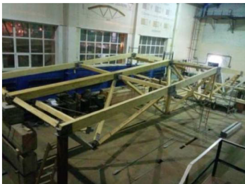
Figure 3. Assembly of a fragment of the structural block: a) the main fabric of the structure; b) 18 × 6 structural block in design position.
