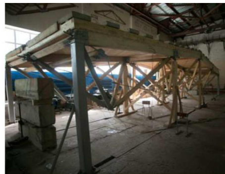
Figure 3. Assembly of a fragment of the structural block: a) the main fabric of the structure; b) 18 × 6 structural block in design position.
